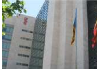
Court Project - Colombia
